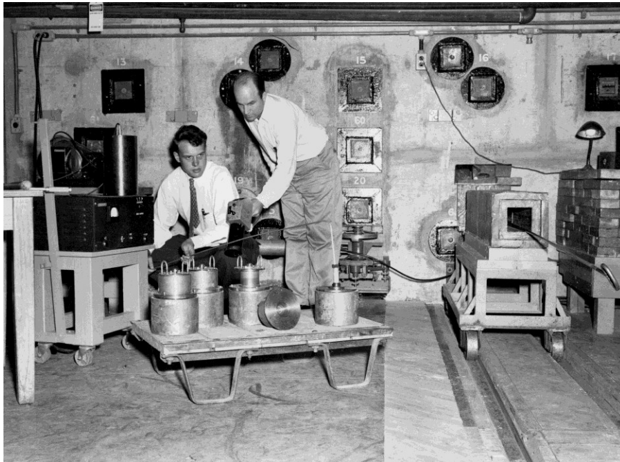
Radioisotopes being carefully removed from the side of the Graphite Reactor
